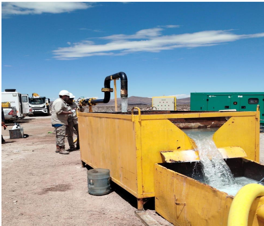
Figure 1. Power’s Incahuasi pumping well progress
